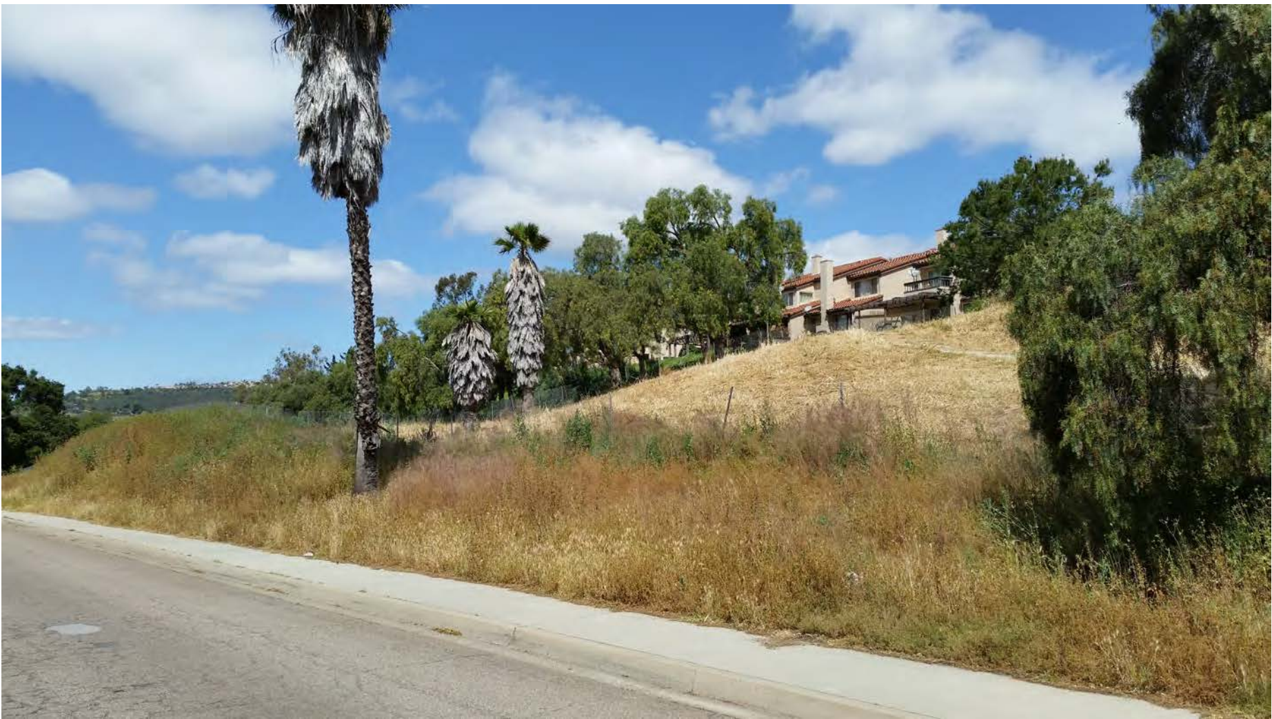
Key View 5 - Existing Conditions
