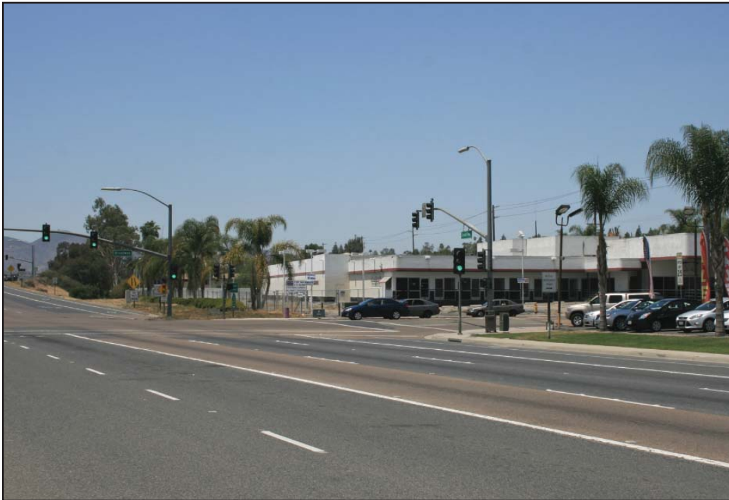
KEY VIEW 1a Existing Conditions: View from East Lincoln Parkway Looking West
