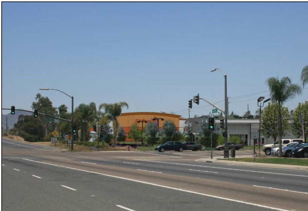
KEY VIEW 1b Proposed Project: View from East Lincoln Parkway Looking West
